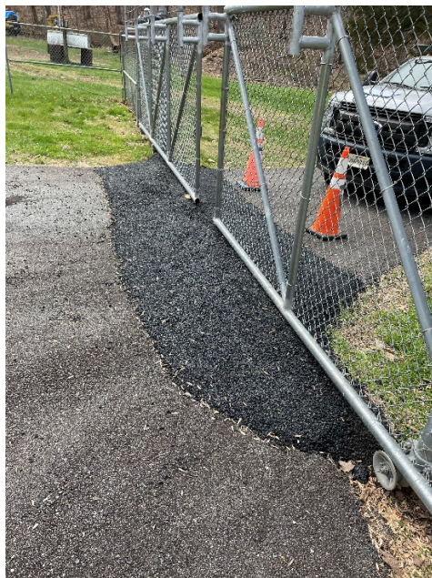
Asphalt Berm at Ashcroft Pump Station No. 1
