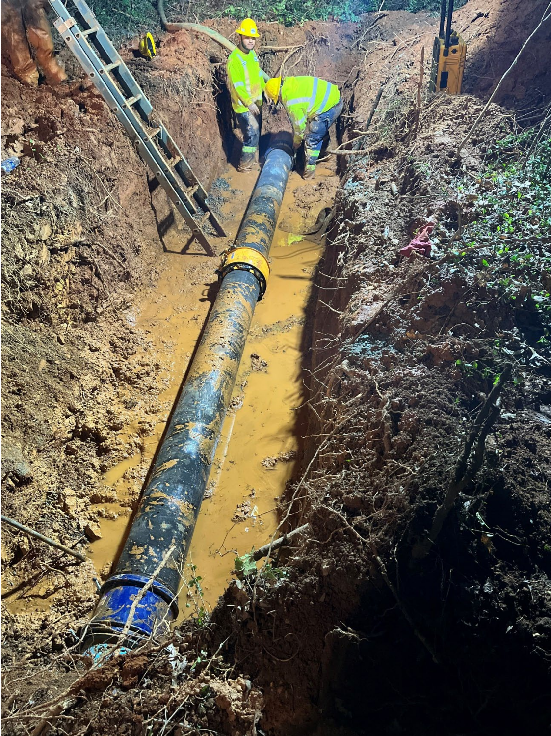
Earlsville Road Water Main Repair – New 12" DIP Water Main: 3/20/24
