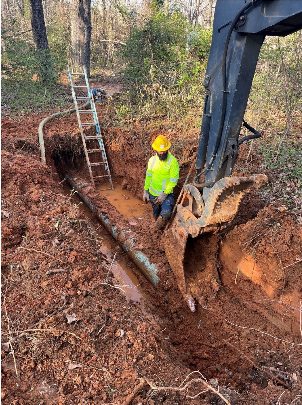
Earlysville Road Water Main Repair – Excavating 12" PVC Water Main: 3/20/24
