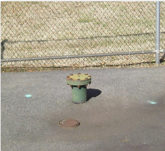
(Attachment 3) Emergency Bypass Connection
