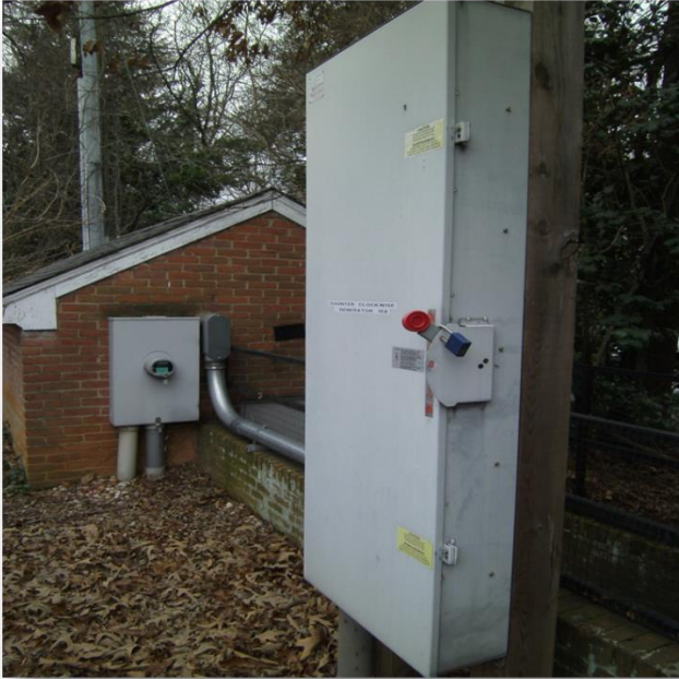
(Attachment 2) Emergency Transfer Switch
