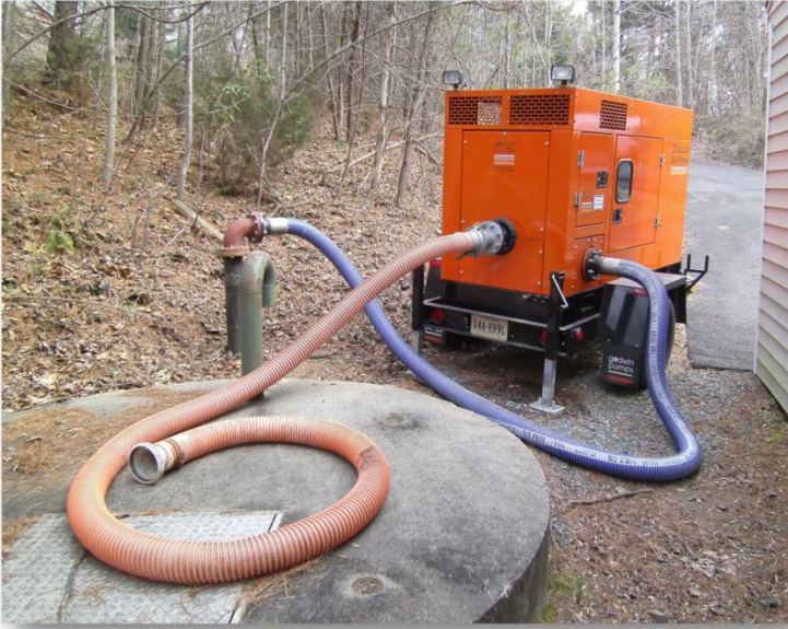
(Attachment 4) Emergency Bypass Pump
