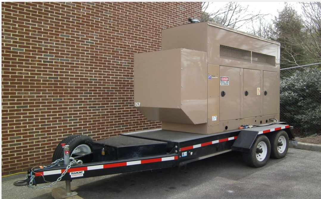
(Attachment 1) Trailer Mounted Generator
