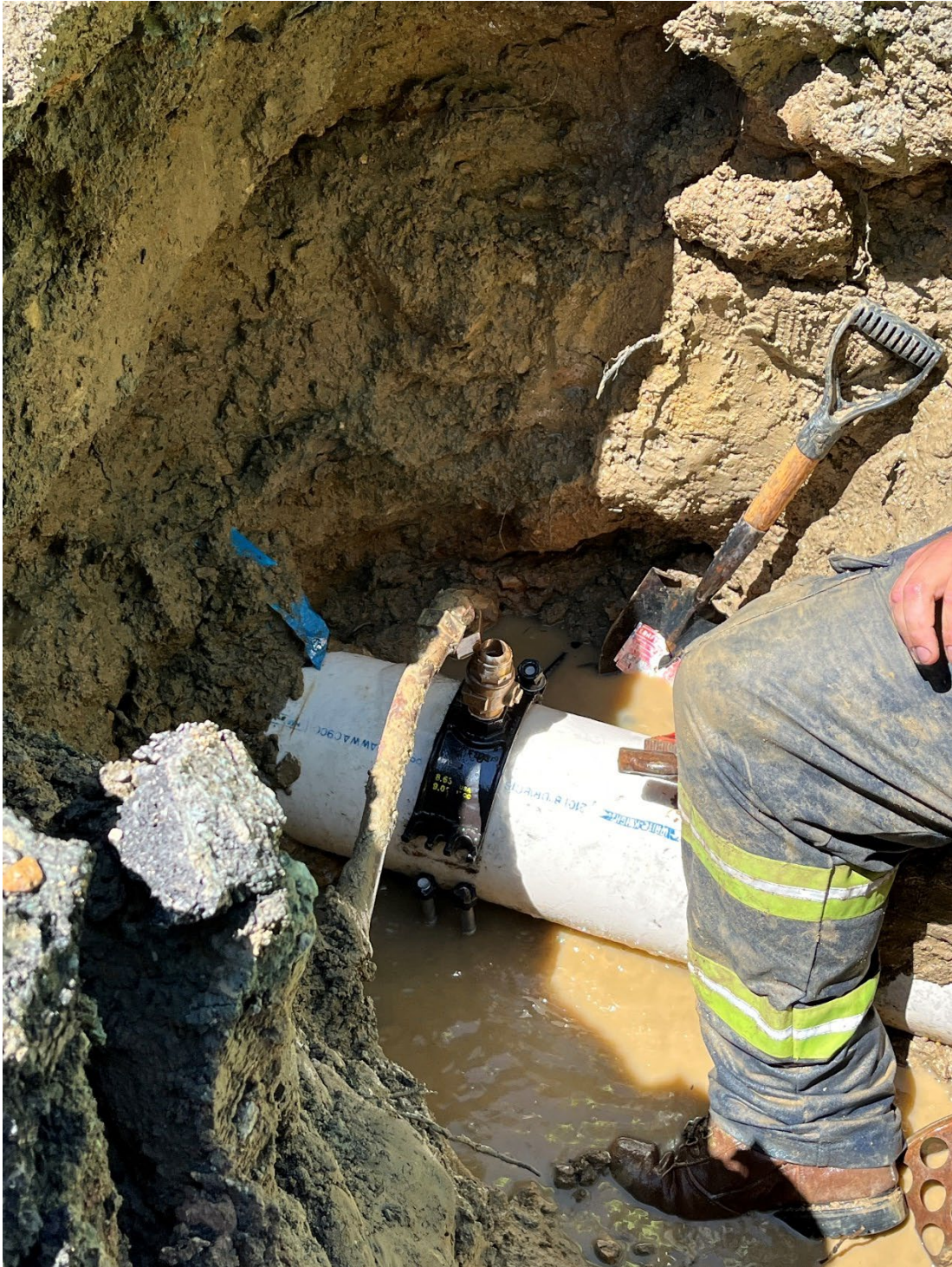
Attachment 2: Townwood Water Leak – Saddle Replacement
