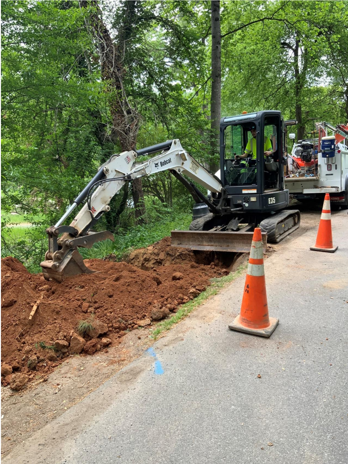
New Water Service Installation – Bellair Subdivision
