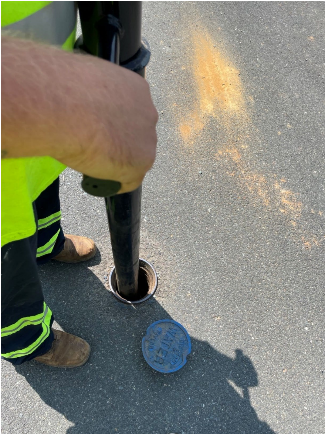
Attachment 4: VAC Excavator Being Used to Clean a Valve Box
