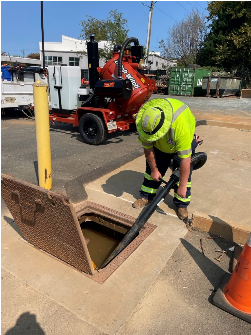
Attachment 3: VAC Excavator Being Used to Clean Vehicle Wash Area Collection Basin
