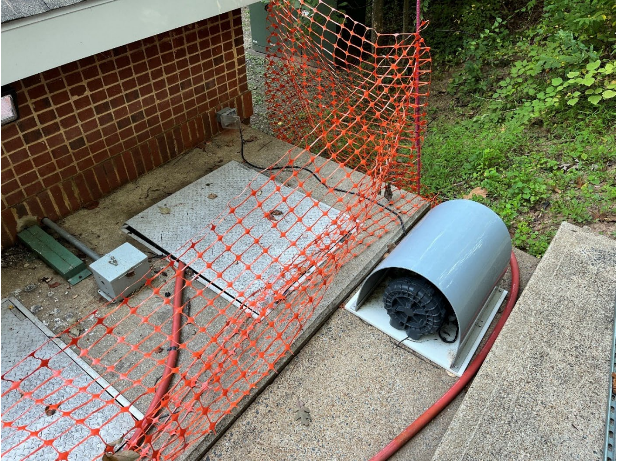
Attachment 1: WetWell Wizard Surface Setup at Old Forge
