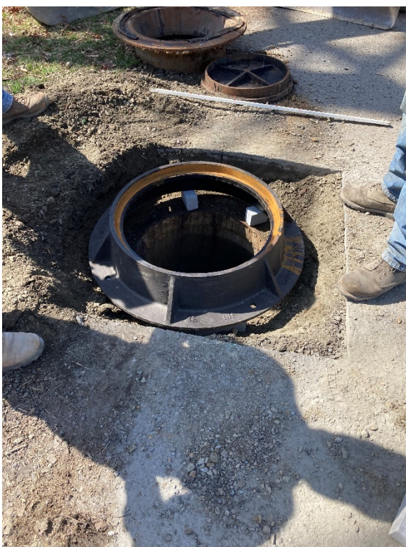
Replace MH Frame and Cover
