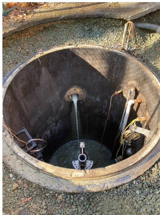
Wet Well with Top Removed
