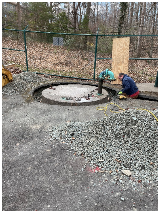
Wet Well with Existing Vault Top
