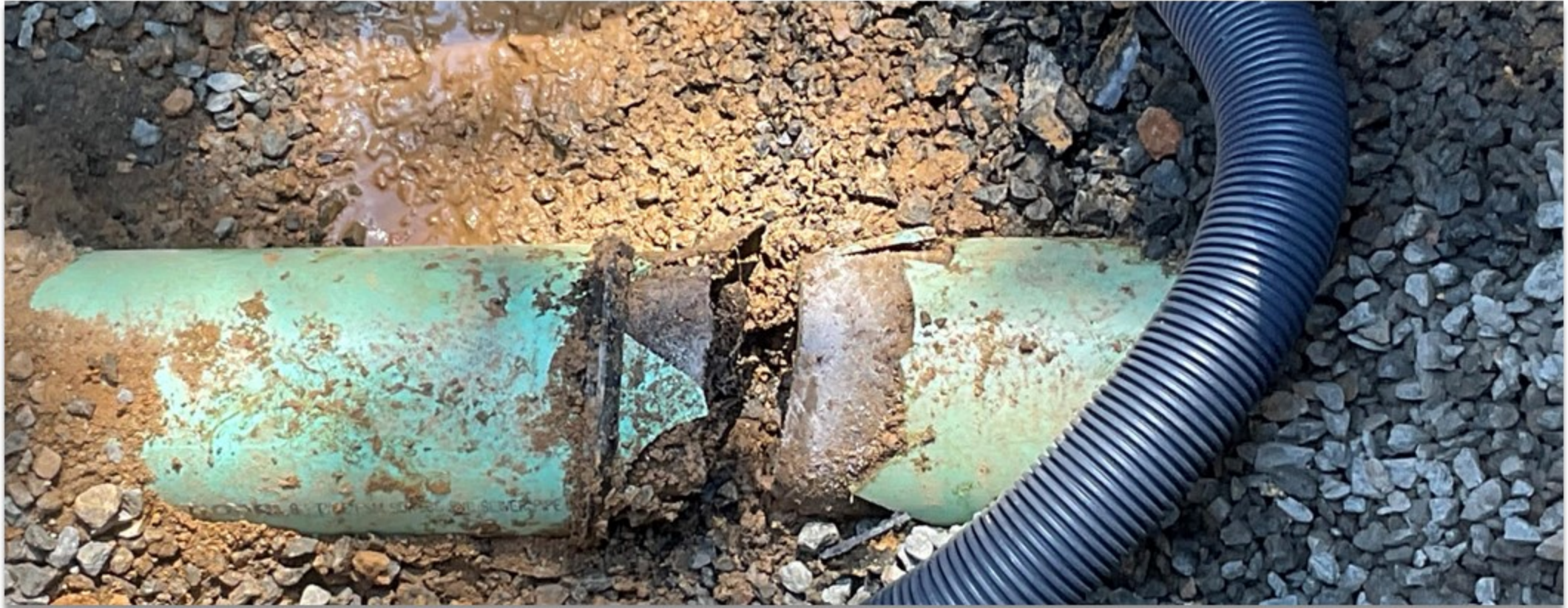
Commonwealth Drive – Utility Line Cable Run Through ACSA Sewer Line
