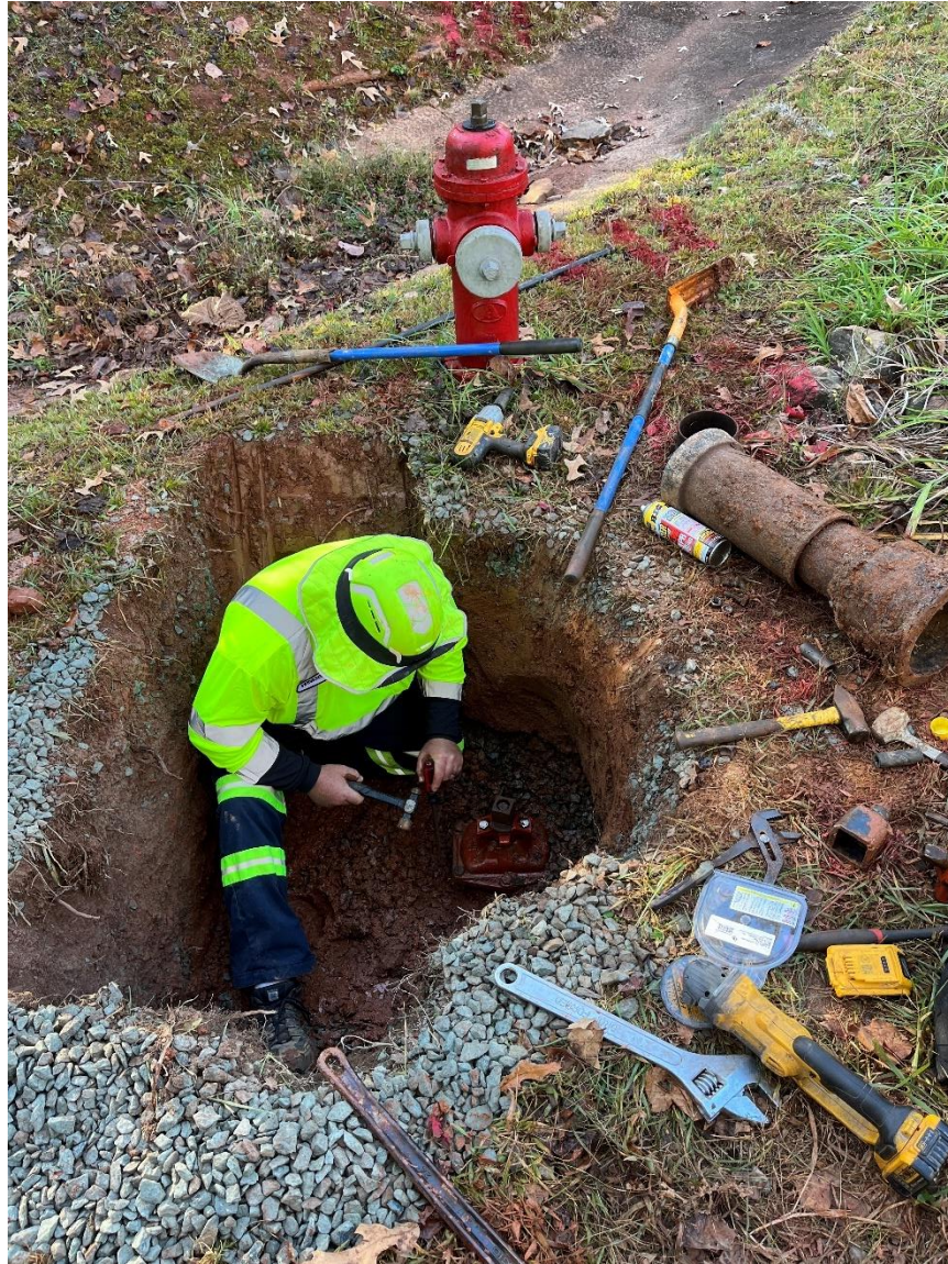
Attachment 8: Fire Hydrant Valve Repair – Key West Subdivision
