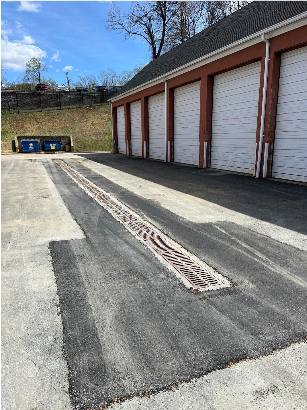
Attachment 6: Maintenance Yard Asphalt Repair
