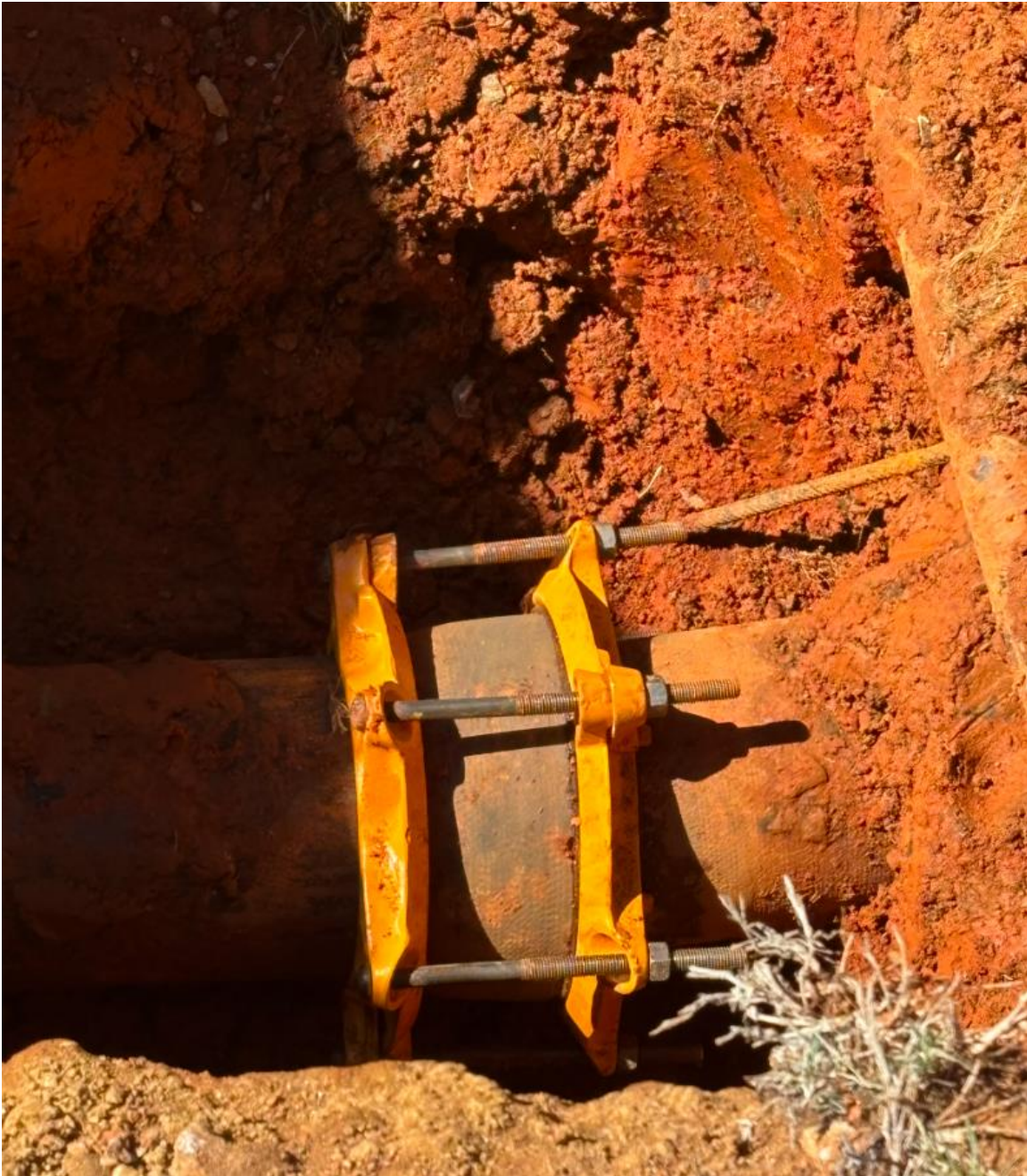
Attachment 1: Verona Drive Water Main Repair
