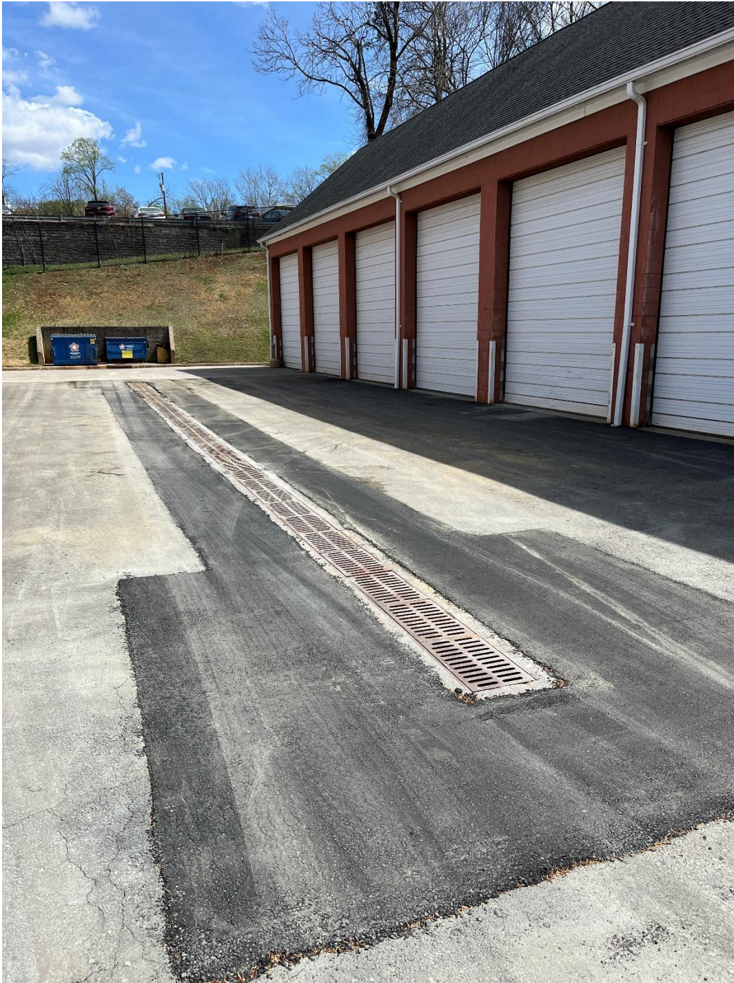
Attachment 6: Maintenance Yard Asphalt Repair
