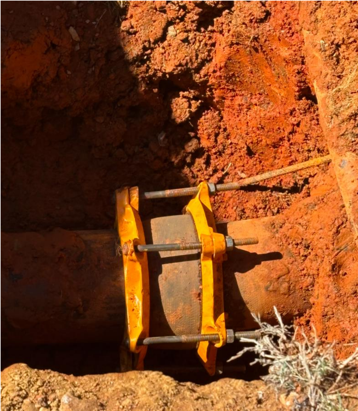
Attachment 1: Verona Drive Water Main Repair
