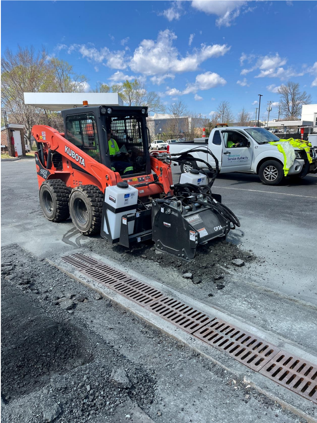
Attachment 3: Erskine 24" Edge Milling Skid Steer Attachment – Picture 2
